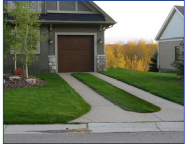
It is always better to allow precipitation to soak into the ground where it falls.
