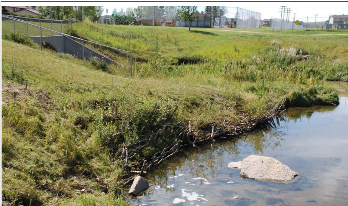
Photo x: Bioengineering techniques (i.e. live willow fences) employed in 2006 remain intact. This photograph taken in 2009 shows that live willow cuttings have helped to stabilise and reshape the bank. There is now reduced erosion along the bank and the willow stems are helping to build out the bank by trapping sediment. Some additional willow fencing may be needed to reinforce this bank as there has been some willow mortality since 2006.
