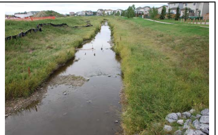
Photo l: Channelization of Nose Creek in Willow Brook Park in Airdrie has caused loss of riparian habitat and may lead to higher downstream erosion. (Photographer: K. Hull, Catalogue Number: RHIP17NOS018).
