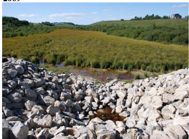
WNO7L Downstream end looking upstream. The wide, robust sedge channel in the middle of the valley persists. Road construction activities have occurred since 2000. A new culvert crossing and associated rip-rap has been installed at this end of the site.
